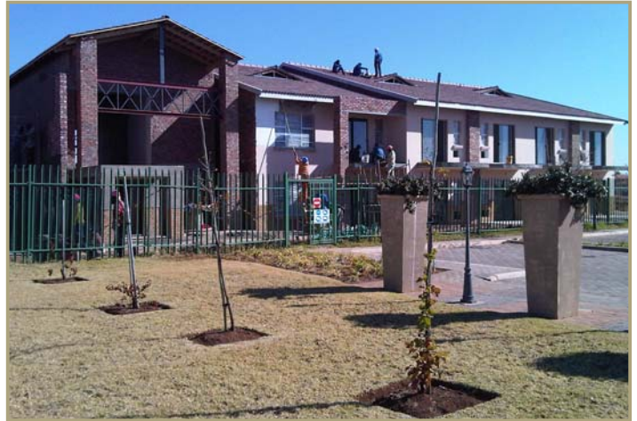
Retreat Apartments Progress - 30 June 2011
